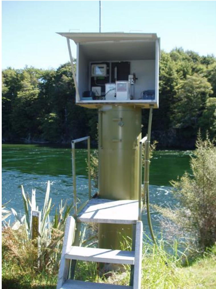
Figure 13 – Typical stilling well housing design.
