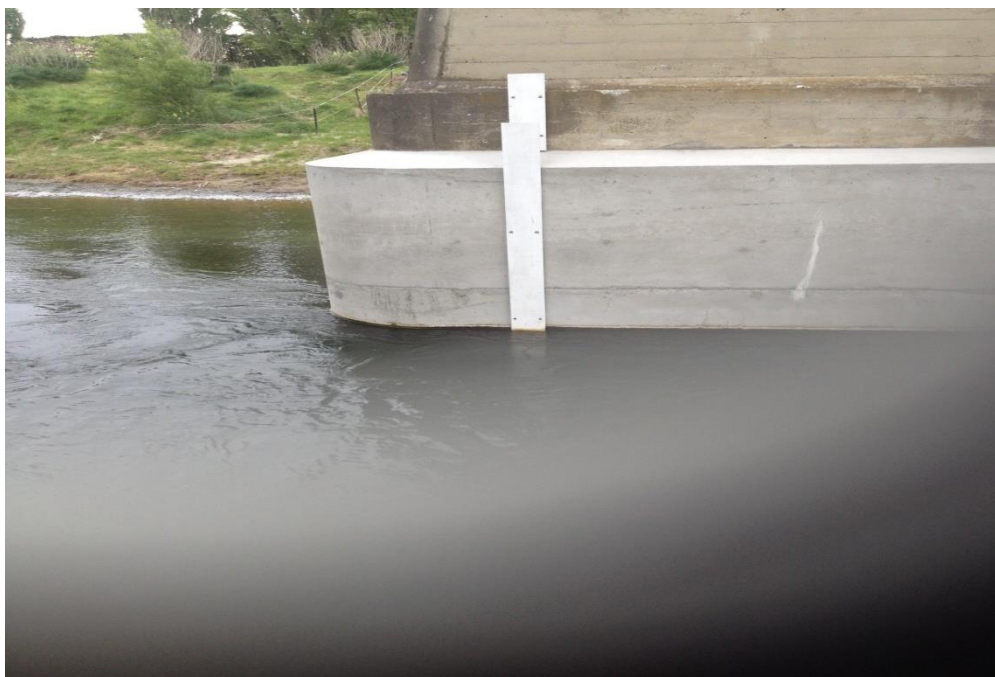
Figure 21 – Timber boards attached to a stable structure
